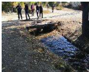
Bridge at PK 26+65
