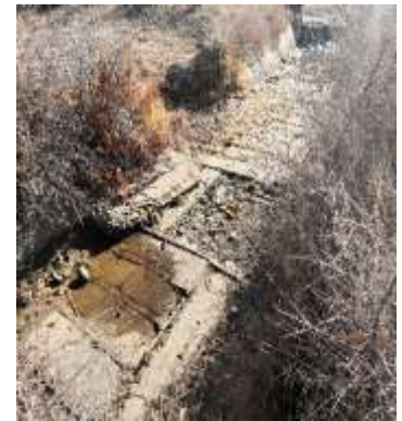
Canal section in slabs
